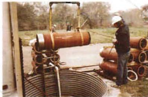
Clay pipe is lowered into jacking pit.
