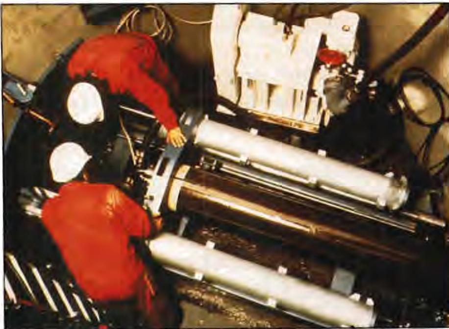
Soltau RVS 100AS microtunneling jacking 12-in. clay pipe.
