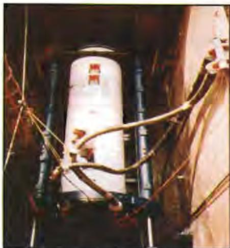
Oscar Renda Contracting's RVS 400A slurry microtunneling machine running on the West Bank Interceptor project, Dallas.
